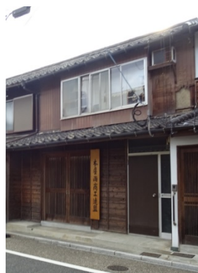
Photo 2. An example that a house is renovated using metal fittings
