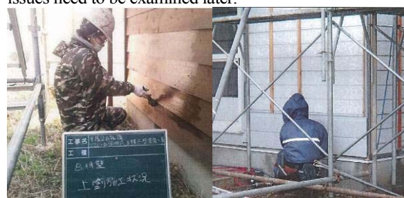
Figure 2. Re-application of protective coating (left) and covering method (right)
