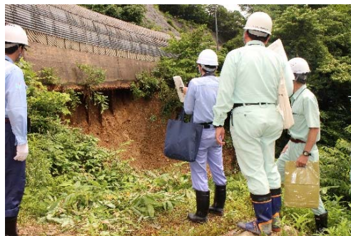
Photo 2: On-site inspection at Noboritani Snow Shelter
