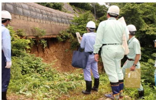
Photo: On-site investigation after the onset of a natural disaster
