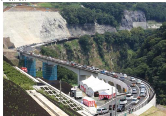
Photo: Resumed service of the Aso Choyou Great Bridge Rout (Aug. 2017)
