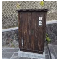
Photo 2 Fire hydrants around the town
