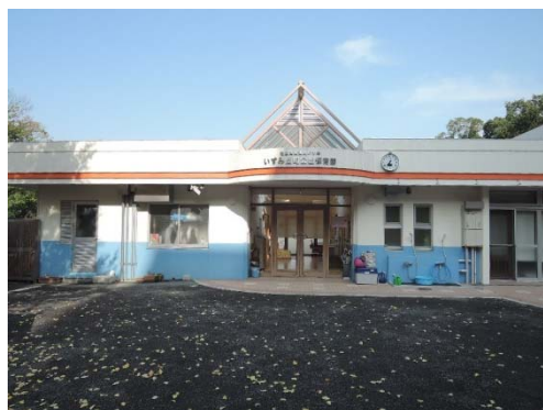
Photo 1: Example of a day nursery installation (Yokohama City Sorimachi Park)
