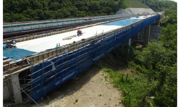
Photo: Tawarayama Bridge under restoration
