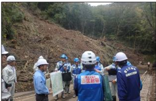
Photo 8 Field survey on National Highway No. 138, Hakone-machi. (Oct. 26)
