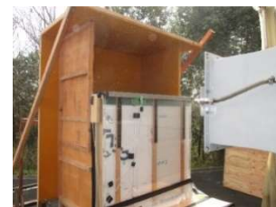
Air blowing and water spraying test on outer walls of ventilation structure
