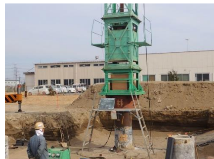
Photo: Vertical load test (rapid loading method)
