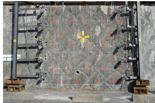
Photo 3: Retaining wall (brick masonry) with which the load test was conducted
