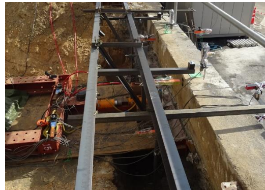
Photo 4: Loading system at the back of the retaining wall
