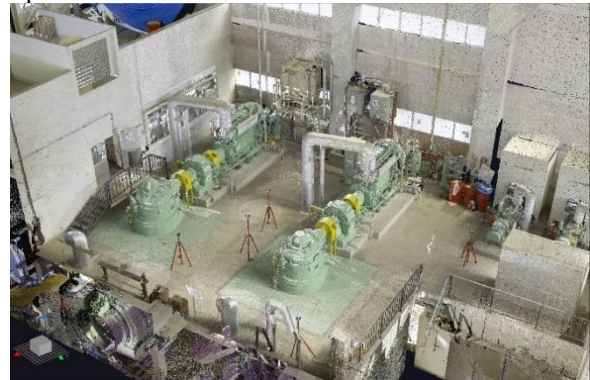
Fig. 1: Point group data of drainage pump stations
