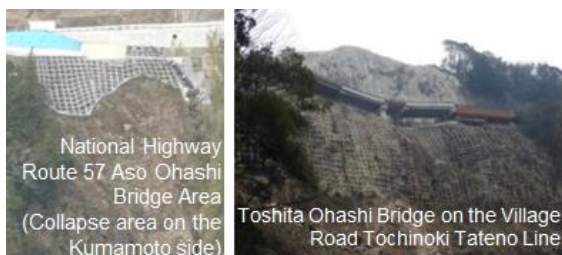
Photo 1: Road close to the steep slope
