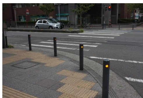
Photo 1: Example of bollard installation (N-type bollard)
