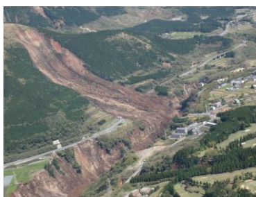
Slope failures caused by 2016 Kumamoto Earthquakes
