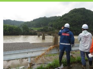
Okitsuru Bridge Survey (July 10)
