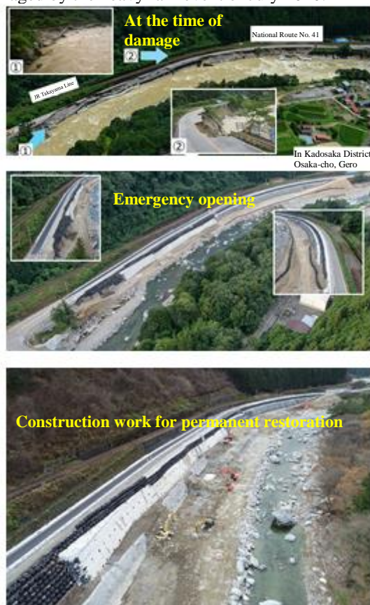
Fig. Photographs of damage to National Route 41 and the state of restoration
