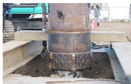
Photo 1: Removal of existing piles in the experiment
