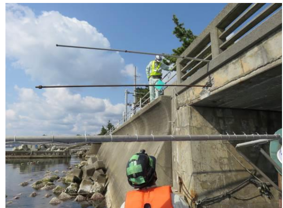
Photo 1: Fracture / protrusion of lateral-fastening PC steel
