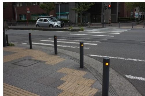
Photo 1: Example of bollard installation (N-type bollard)
