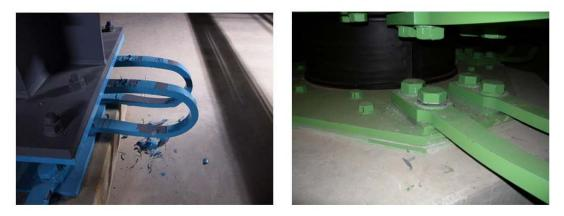
Photo 9.2-22 Peeling off of paint and loose of the bolts of U-shaped steel dampers
