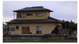
Photo 6.2-71 Falling down of mortar plastered wall
