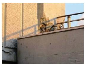
Photo 6.3-21 Crushing at the bottom of column of the multi-story shear wall
