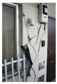
Photo 6.3-30 Shear cracks on nonstructural wall
