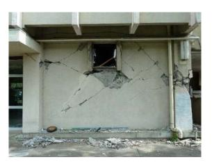
Photo 6.3-19 Shear failure of wall with opening
