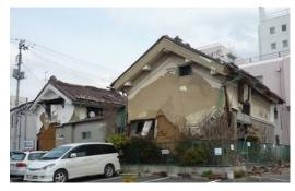
Photo 6.2-47 Failed warehouse with mud wall
