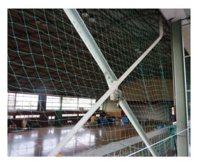
Photo 6.4-1 Buckling of brace
