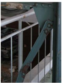
(a) Latticed column (b) Buckling of diagonal member Photo 6.4-5 Buckling of diagonal member of latticed column
