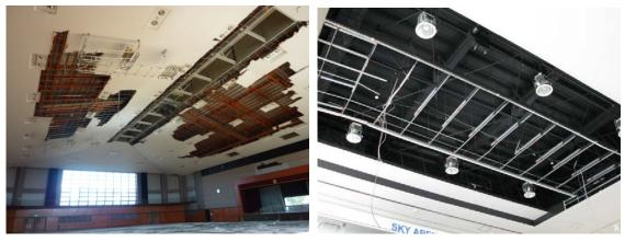
Photo 6.6-15 Falling of metal furring suspended ceiling
