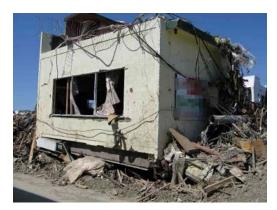
Photo 7.2-1 Story collapse of a 2-story reinforced concreted building
