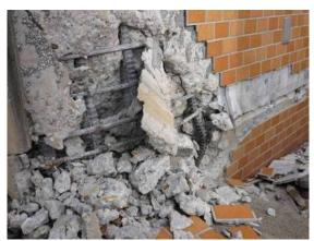
Photo 6.3-23 Damage at the bottom of SRC column
