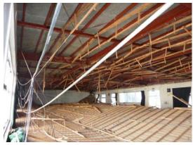
Photo 6.4-17 Dropping of extensive ceiling components
