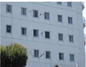
Photo 6.3-46 Shear crack on nonstructural wall
