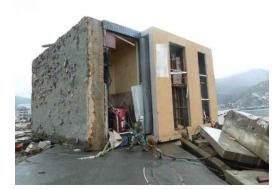
Photo 7.2-2 Overturning of a 3-story reinforced concrete building
