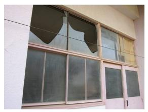
Photo 6.6-9 Breakage of window glasses installed to fixed window frame with hardening putty
