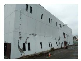
Photo 7.2-5 Out-of-plane fracture of reinforced concrete shear wall without floor
