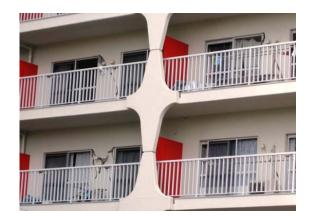
Photo 6.3-31 Shear cracks on mullion
