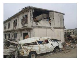
Photo 7.2-6 Wall opening generated by debris impact
