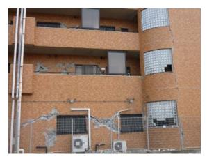
Photo 6.3-43 Damage of nonstructural wall in same building shown in Photo 6.3-22
