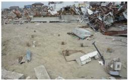
Photo 7.4-11. Steel tube pile left at the the original position (2) of photo 7.4-10.
