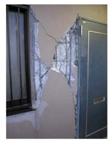
Photo 6.3-42 Shear failure of nonstructural wall
