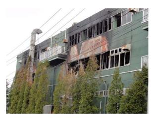
Photo 8.3-2 Fire scene at a factory building (Oushu city, Iwate prefecture)
