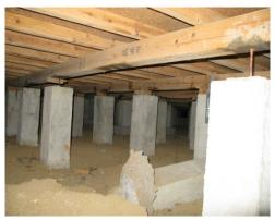
Photo 6.4-13 Overturning of floor strut
