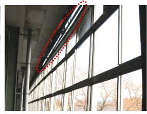
Photo 6.6-12 Breakage of glass mullion of Photo 6.6-13 Dislocation of window frame glass wall system
