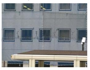
Photo 6.3-49 Damage of tile on exterior wall
