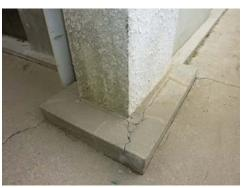
Photo 6.4-12 Cracking of column base concrete
