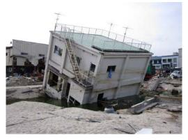
Photo 7.2-4 A 2-story reinforced concrete building that was tilted by scouring
