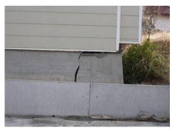
Photo 6.2-67 Crack of foundation
