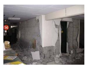
Photo 6.3-16 Failure of shear wall
