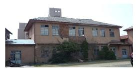
Photo 6.2-17 School building suffering damage on roof tiles and exterior walls
