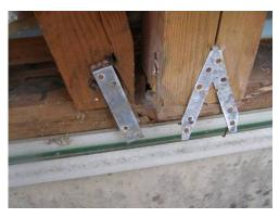
Photo 6.2-59 Metal fastener at the end of column and brace
