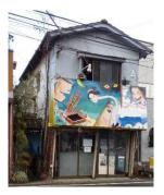
Photo 6.2-41 House with large residual deformation (Komatsujima)
