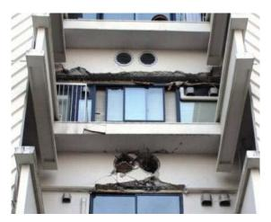
Photo 6.3-28 Damage of boundary beam with opening
