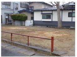
Photo 6.2-2 Sand boil due to liquefaction
