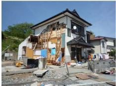
Photo 7.4-27. Wood house ([]) remained under the flood water depth of over 7 m in Akasaki-cho, Oofunato city.
