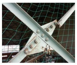
Photo 6.4-2 Net section fracture at bolt hole
