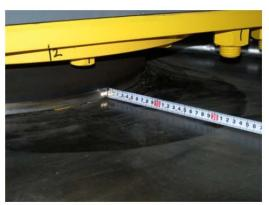
Photo 9.2-24 Trace of displacement of elastic sliding bearing
