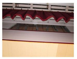
Photo 6.6-23 Falling of cement mortar finish above stage
