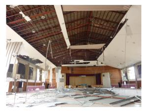
Photo 6.4-18 Dropping of extensive ceiling components
