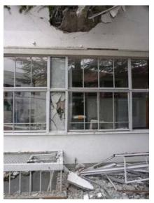
Photo 6.3-8 Shear failure of the first-story column
