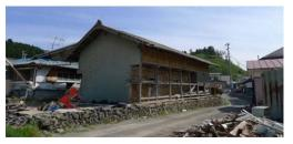
Photo 7.4-32. Survived soil warehouse (10) which seemed to have comparatively slight structural specifications in Akasakicho, Oofunato city.
