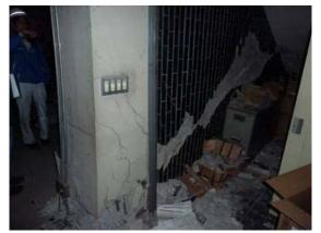
Photo 6.3-10 Shear crack on shear wall
