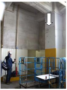
Photo 9.2-7 Trace of tsunami water
