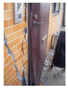
Photo 6.3-44 Damage of nonstructural wall and deformed door in same building shown in Photo 6.3-22
