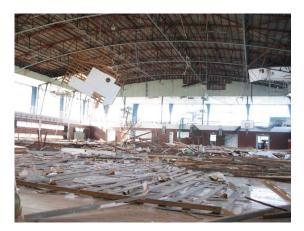
Photo 6.6-14 Falling of wooden suspended ceiling
