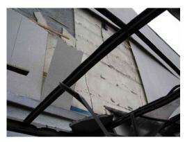
Photo 6.4-20 Falling of exterior finish components
