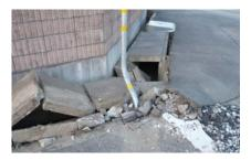
Photo 6.5-6 Damage of side ditch
