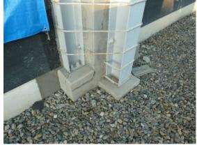
Photo 6.3-11 Column strengthened with H-shaped steel
