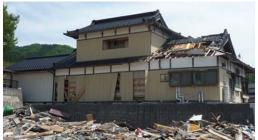
Photo 7.4-30. Wood house (6) which was not carried away in spite of damage on 1<sup>st</sup> floor roof system in Akasaki-cho, Oofunato city.
