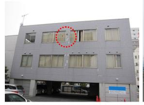
Photo 6.6-6 Falling of ceramic wall tiles and breakage of AAC panels
