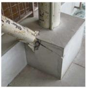
Photo 6.4-11 Cracking of column base concrete
