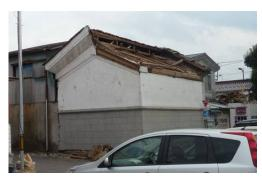
Photo 6.2-48 Fallen roof of warehouse with mud wall
