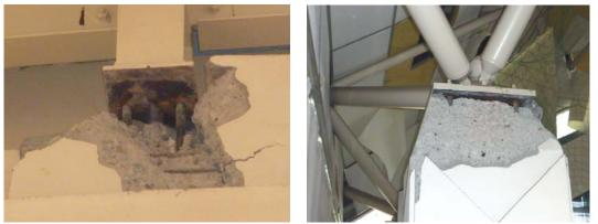
Photo 6.4-6 Spalling of concrete
