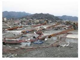
Photo 7.2-8 First-floor columns falling in the same direction
