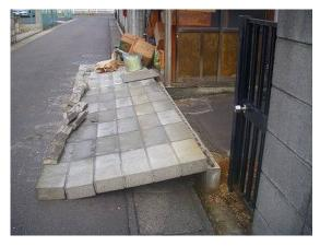
Photo 6.3-50 Collapse of concrete block wall (Koriyama city)
