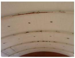
Photo 6.4-14 Peeling of paint of beams
