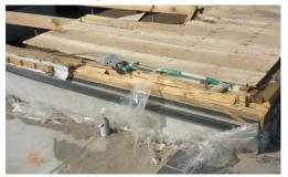
Photo.7.4-4. Sills, foundations and floor boards remained.
