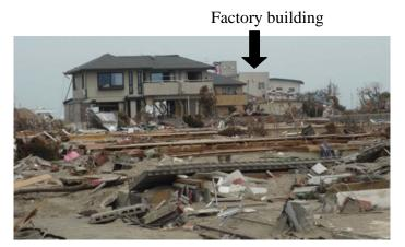
Photo 7.4-21. Wood house (15) which were not washed away selectively in the downstream of a factory building.
