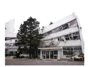
Photo 6.3-7 Mid-story collapsed building (Fukushima city)
