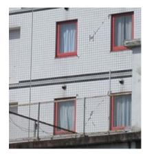
Photo 6.6-1 Detachment of ceramic wall tiles from damaged RC exterior wall
