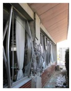
Photo 6.3-15 Shear failure of short column
