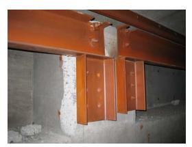
Photo 6.4-8 Pullout of hole-in anchors
