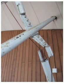
(a) Fracture at column top(b) Fracture at brace crossingPhoto 6.4-3 Fracture of brace welded connection
