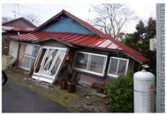
Photo 6.2-3 Damage of houses caused by ground transformation
