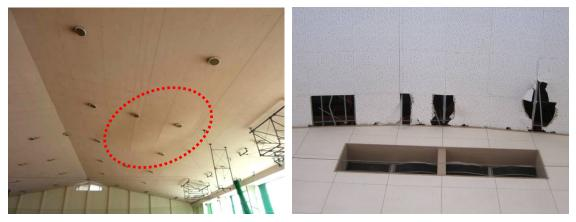
Photo 6.6-19 Sagging of metal furring suspended ceiling
