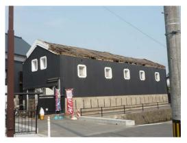
Photo 6.2-12 Warehouse with mud walls whose roof system with roof tiles fell down
