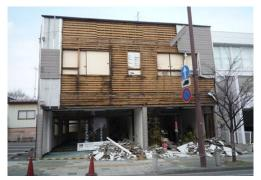
Photo 6.2-44 Fallen mortar of wall (Wood house with store)
