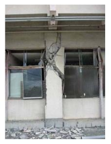
Photo 6.3-18 Shear failure of column
