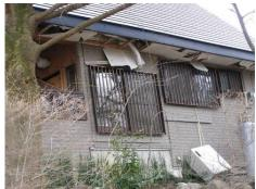
Photo 6.2-61 Failed ceiling of eave
