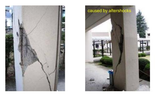
Photo 6.3-13 Shear cracks of first-story columns
