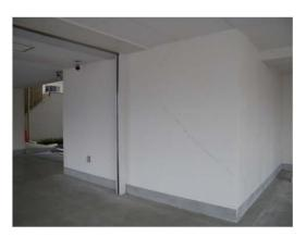
Photo 9.2-14 Shear crack on the wall
