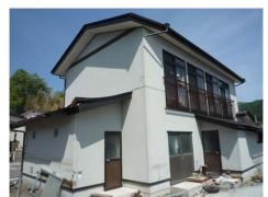
Photo 7.4-28. Wood house (3) without damage under the flood water depth of over 7 m in Akasaki-cho, Oofunato city.
