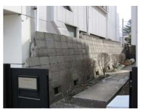
Photo 6.3-51 Collapse of concrete block wall (Sukagawa city)
