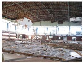
Photo 6.4-16 Dropping of extensive ceiling components
