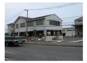
Photo 9.2-8 Tsunami damage to surrounding buildings
