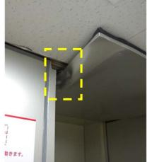
(a) Damage to the panel (b) Damage to the expansion joint Photo 9.2-2 Damage near the boundary between isolated and non-isolated floors
