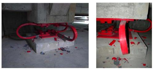
(a) Peeling off of paint (2) Deformation of steel Photo 9.2-19 Deformation of U-shaped steel damper
