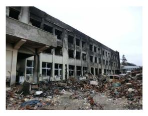
Photo 8.2-1 Tsunami fire at an elementary school (Ishinomaki city, Miyagi prefecture)
