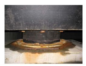
Photo 9.2-10 Rust of High-damping rubber bearing
