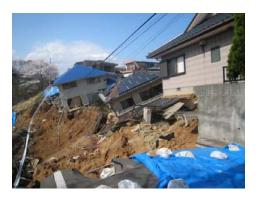
Photo 6.5-18 Land sliding of slope on the southwest of hill and sliding houses
