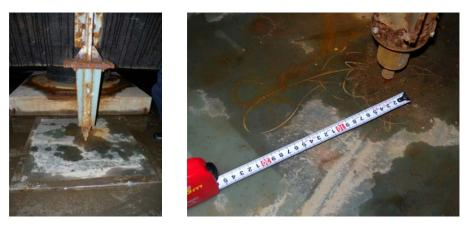
Photo 9.2-11 Trace of displacement of the SI floor on the scratch board
