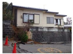
Photo 6.2-37 Damage of retaining wall and houses (Oritate, Aoba ward)
