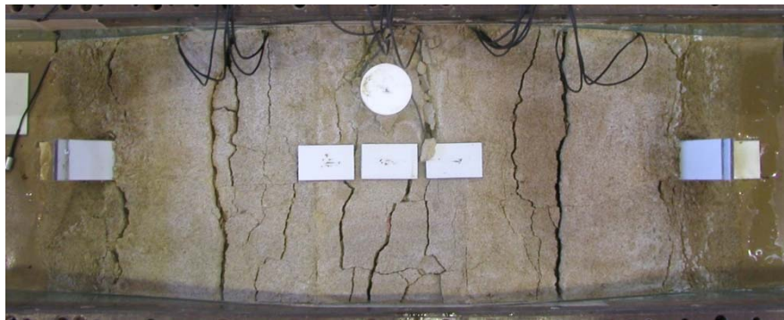
天端沈下0.75m
