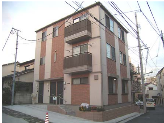
写真 道路斜線制限等の緩和を受け総3階で建替った建物の例（東京都品川区戸越一丁目） Fig. An example of a building rebuilt with 3 full stories with a variance of height controls to a front road, and so on (1-chome, Togoshi, Shinagawa Ward, Tokyo)
