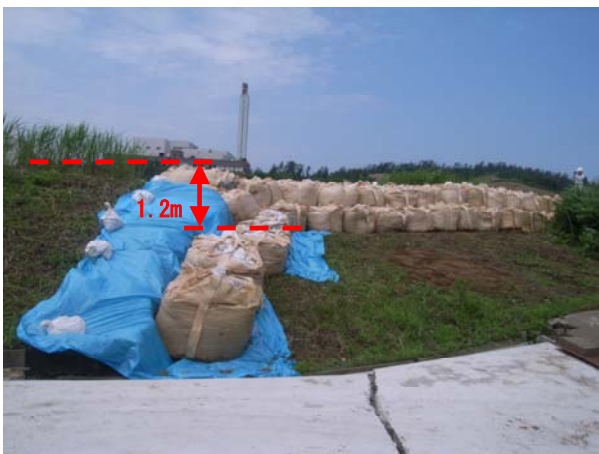
写真-2 鯖石川2kp付近左岸の横断亀裂を伴う沈下 Photo 2. Settlement caused by lateral cracking on the left bank near 2kp on the Sabaishi River
