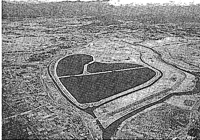
Watarase Retarding Basin (Construction began in 1911)
