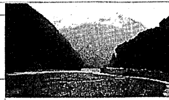
Partially, riverbed aggradation of more than 100m after the earthquake
