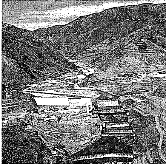
Ashio Sabo Dam (Watarase River)
