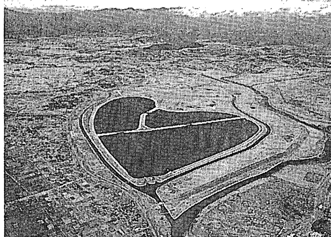
Watarase Retarding Basin (Construction began in 1911)
