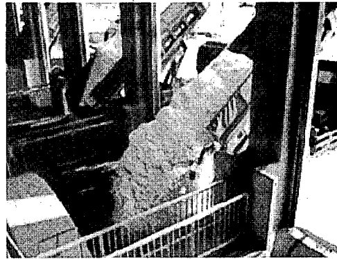
Fig.9 Snow-melting tank using sewerage facilities
