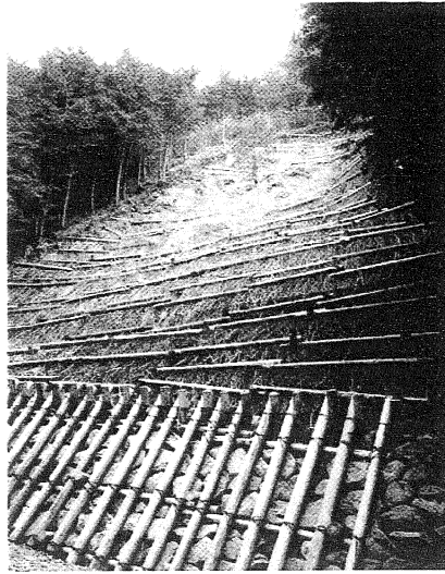
Tsuchiyabara hillside work: Early stage of execution in 1989
