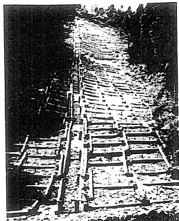
Immediately after completion (1989)
