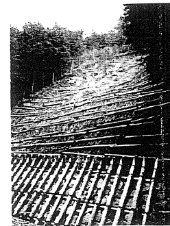
Immediately after completion (1991)
