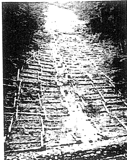
One year after completion (1990)
