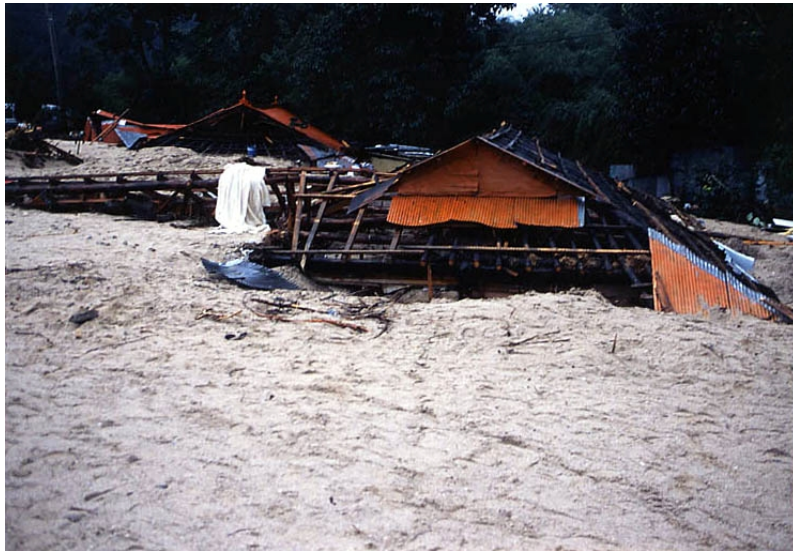
Figure 12. Houses buried by debris flow
