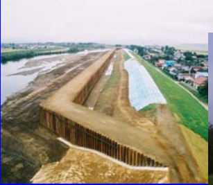
Emergency recovery construction
