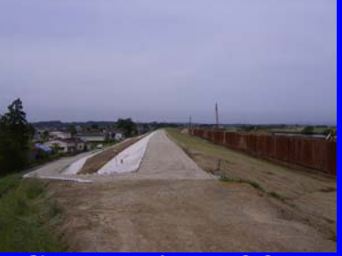
Completion of full recovery construction
