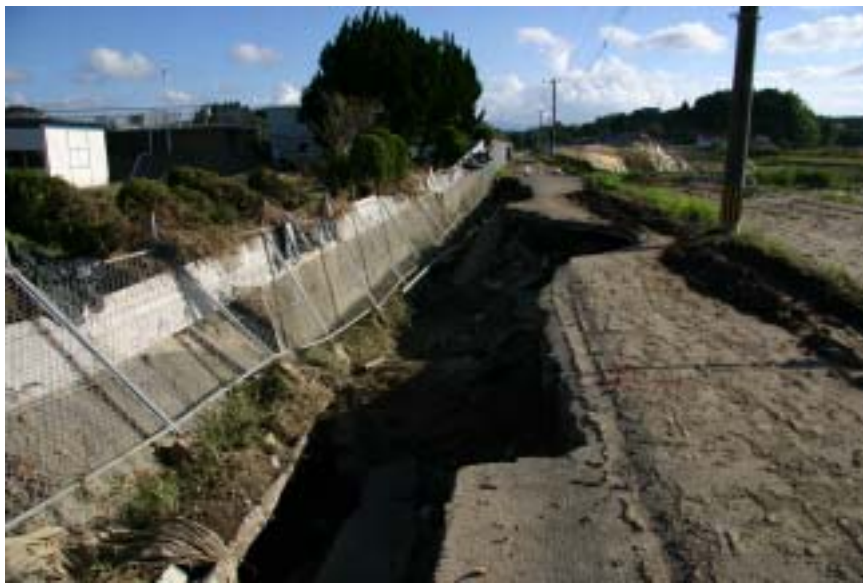
Damage of facility for drinking water in MIYAZAKI city
