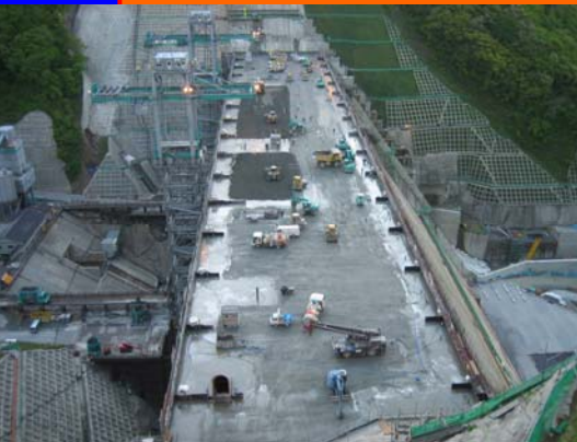
Nagai Dam (in construction)
