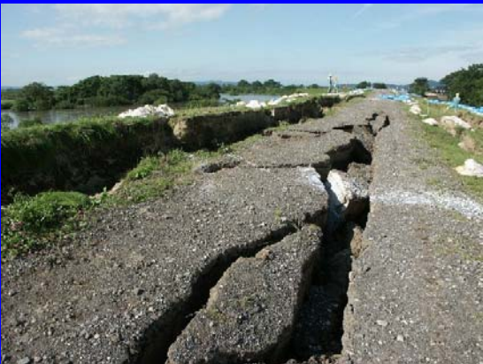
Vertical crack at the edge of weir top
