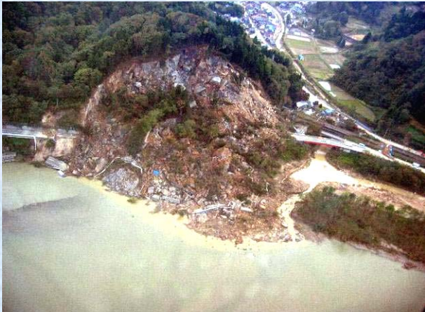
The full view of the slope failure site. This disaster attacked across a 200 m long portion of the road.
