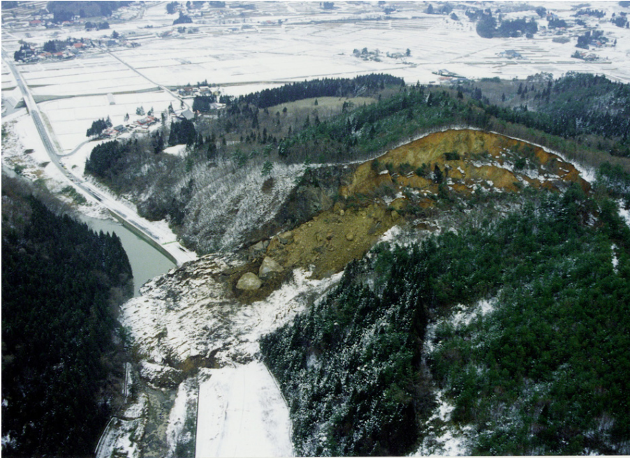
Aerial photograph of landslide
