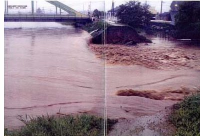
Increasing flood damage (2004)
