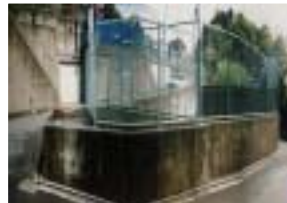
Former flood control reservoir (of a capacity level of approximately 500m 3 )
