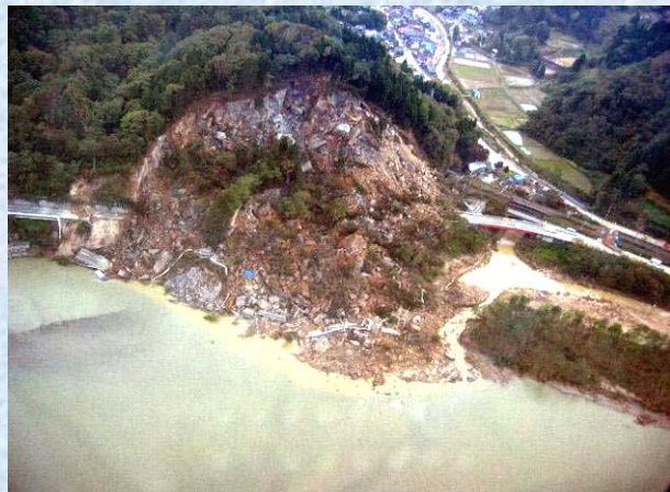
The full view of the slope failure site. This disaster attacked across a 200 m long portion of the road.
