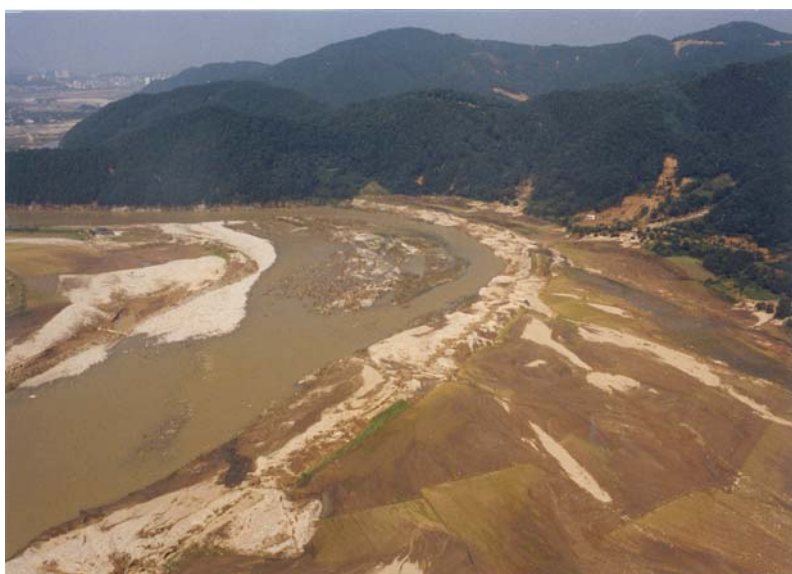
Figure 11. Levee failure, channel widening and recouring (flow from center-left to lower-left)
