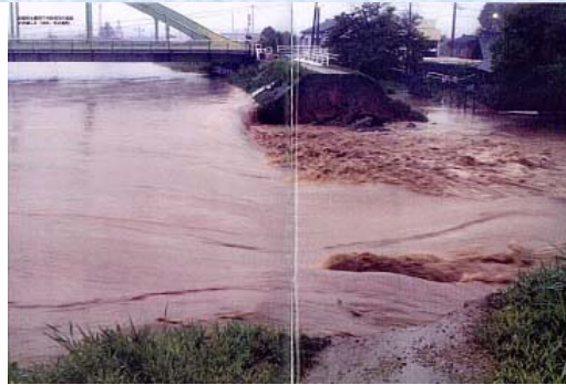
Increased number of floods in 2004: Broken at six points of the Kariyata- river embankment, Niigata
