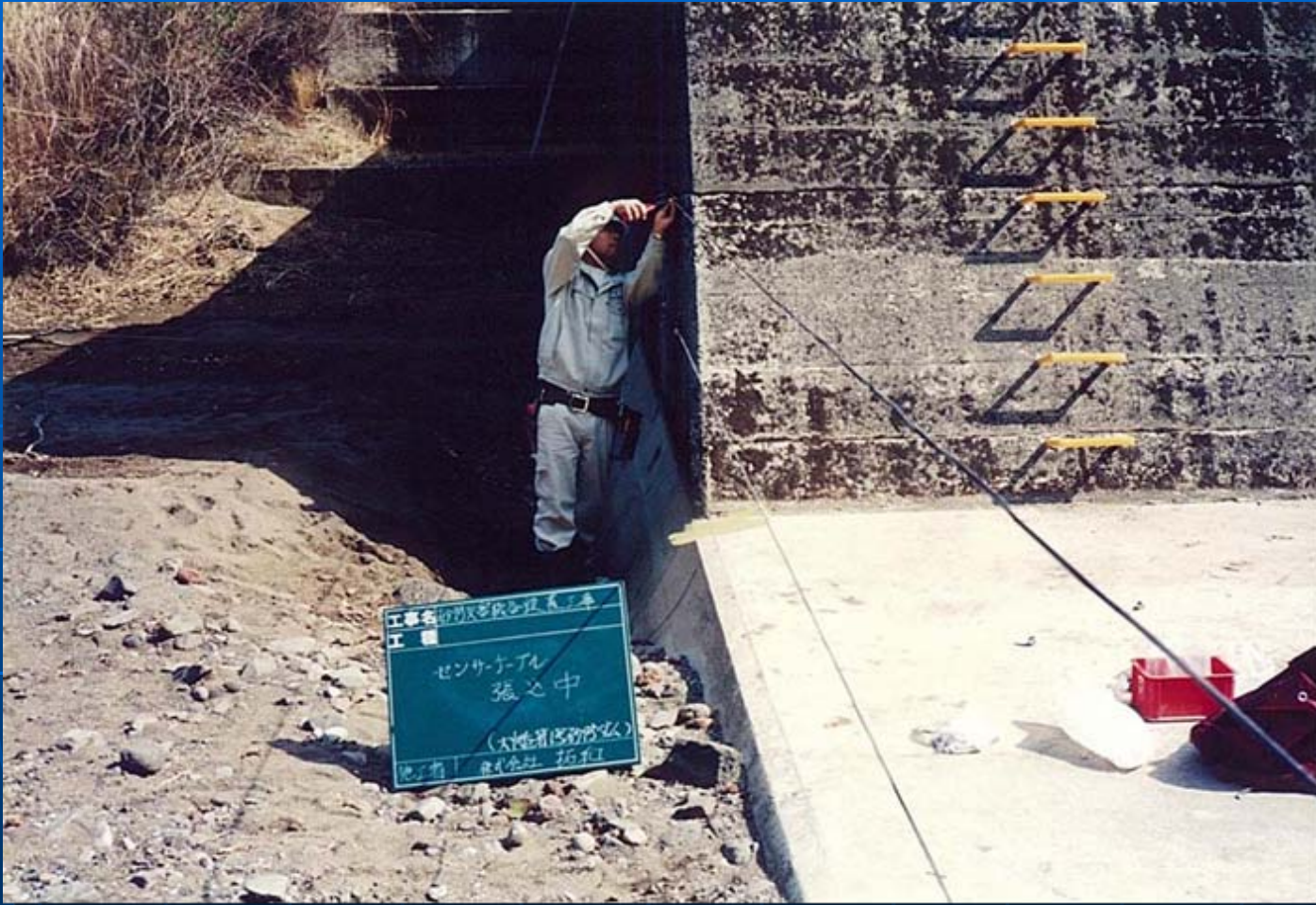
Sensor Being Installed
