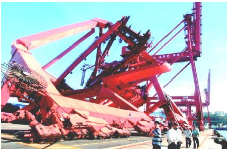
Figure 14. Container cranes destroyed in Busan Port
