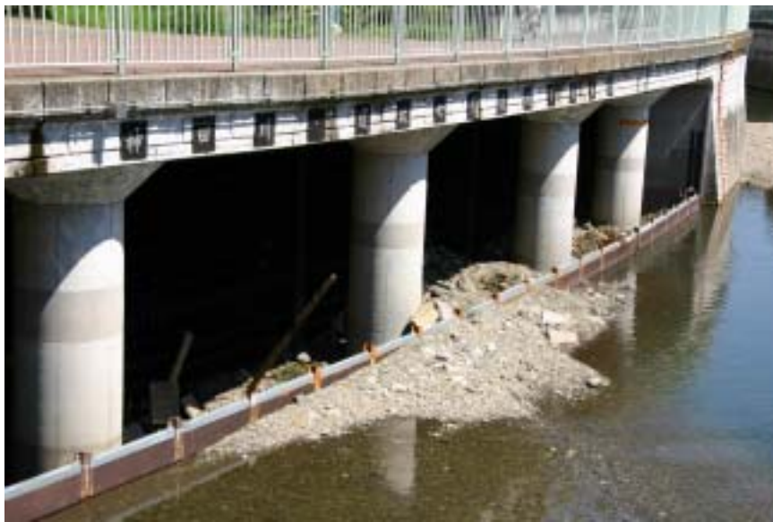
Entrance of underground spill way in TOKYO
