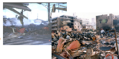
火災被害の例 Example of damaged buildings by a fire
