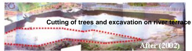
Control of discharge capacity (image)
